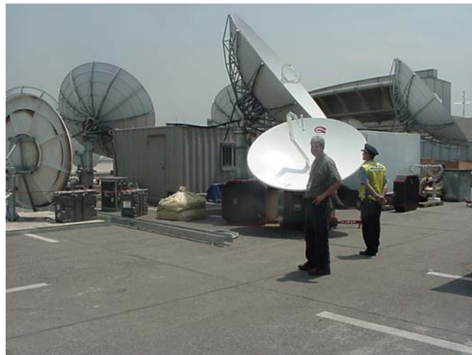
Enliten's Michael Howe inspects Antennae on the roof of the Media Center
